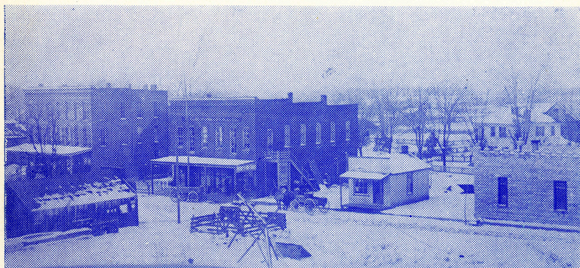
View of Bethalto Business District About Fifty Years Ago
