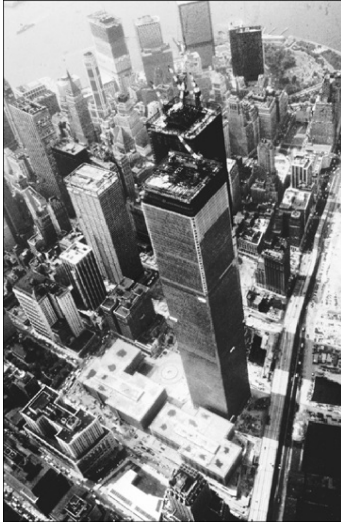
The Twin Towers of the World Trade Center near completion in July 1971. This project marked the culmination of Wall Street's redevelopment, which began when Chase decided to locate its new headquarters downtown. The old elevated West Side Highway runs along the base of the towers, and at the extreme right is the fill from the World Trade Center, upon which the World Financial Center would rise in later years. (Photo by the Downtown-Lower Manhattan Association; courtesy of the Rockefeller Archive Center)
